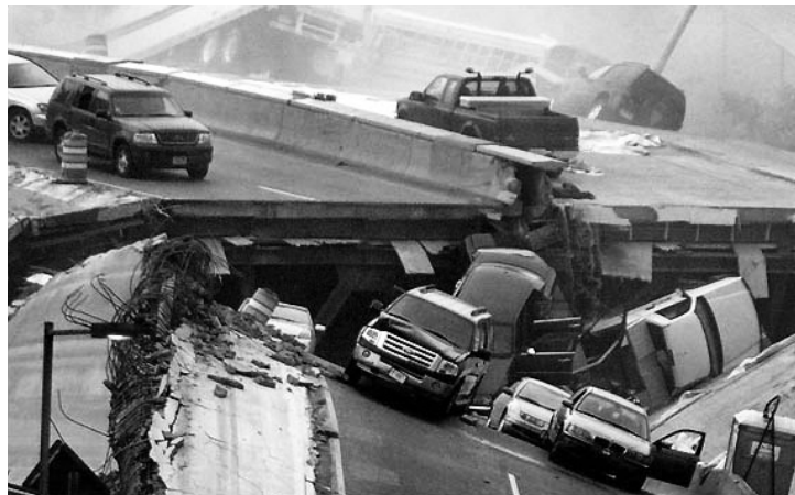
In August 2007, the collapse of the eight-lane bridge in Minneapolis carrying Interstate-35W over the Mississippi River took the lives of 13 people and injured more than 100 others.
