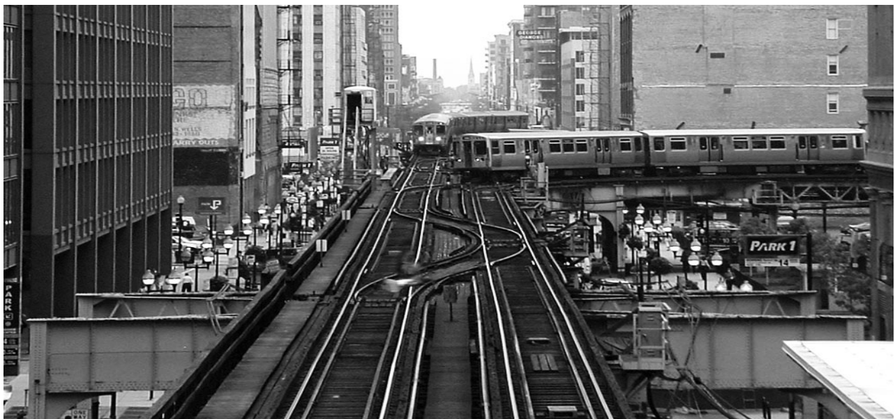
A Brown line train and Orange line train contend for the intersection at the southeast corner of the Loop in Chicago.
