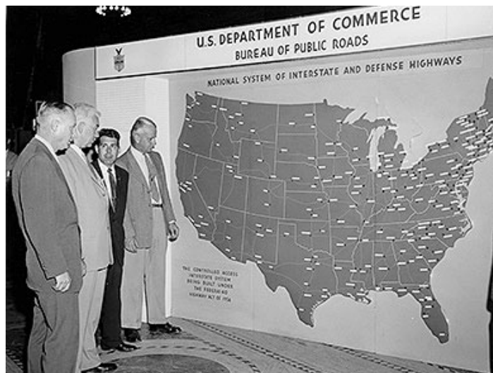
The Bureau of Public Roads developed an exhibit in 1957 — one of many over the years — to let the public know about the “controlled access Interstate System being built under the Federal-Aid Highway Act of 1956.” LEFT TO RIGHT, Robert M. Monahan, special assistant for public affairs; Federal Highway Administrator Bertram D. Tallamy; Harold C. Wood, Sr., of the Motion Picture and Exhibits Section; and Assistant Commissioner for Research E. H. “Ted” Holmes.
