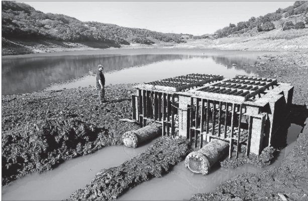
Jerry Sparkman of the Santa Clara Water District stands near the intake structure at Chesbro Reservoir in Morgan Hill. The structure is normally underwater, but not after three years of severe drought.
